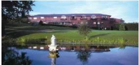
Extension to Hotel at Hill Valley Golf Club, Whitchurch
