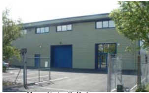
Marine Centre, Pwllheli
